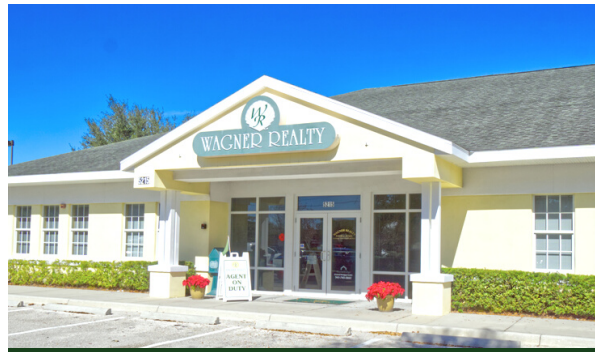
SR 64 East Office Bradenton
